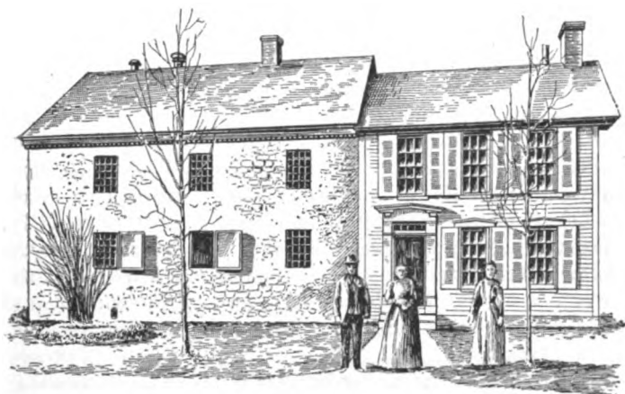
COUNTY JAIL, USED FROM 1839 TO 1894.
